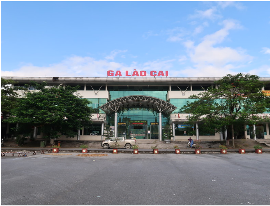
Lao Cai-Hanoi-Hai Phong Railway
